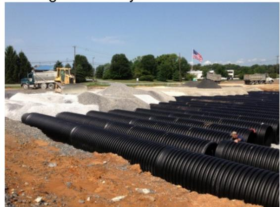
The detention systems, located in the front and the back of the property, were installed by JVH Excavating (Lemoyne, PA.). Excavation area measured 158 x 246 feet for the 48 inch
